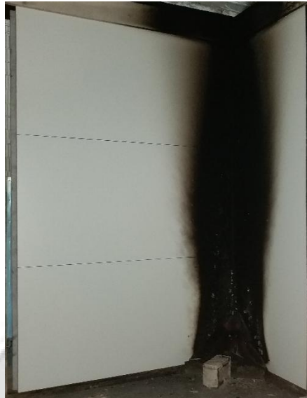
Plate 3: At end of test
